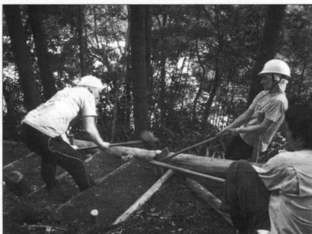
Figure 4. Thinned conifer trees utilized to construct nature trail in Kurogi, Fukuoka.
